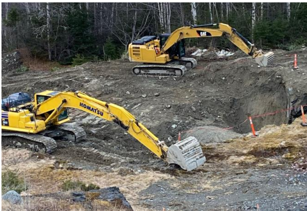
Figure 7: Start of Penstock Excavation
