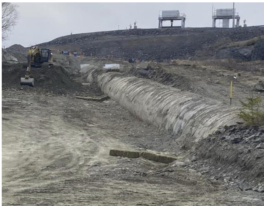
Figure 8: Excavation of First 100 m – Cans 2-8
