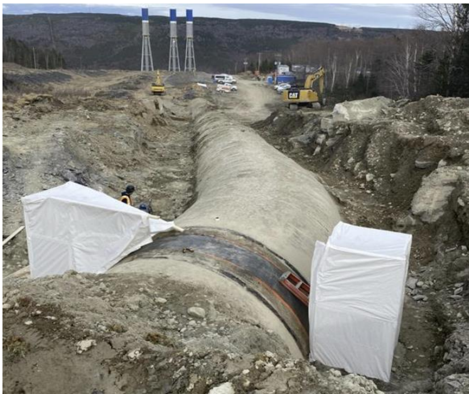
Figure 9: Asbestos Abatement Cut 1
