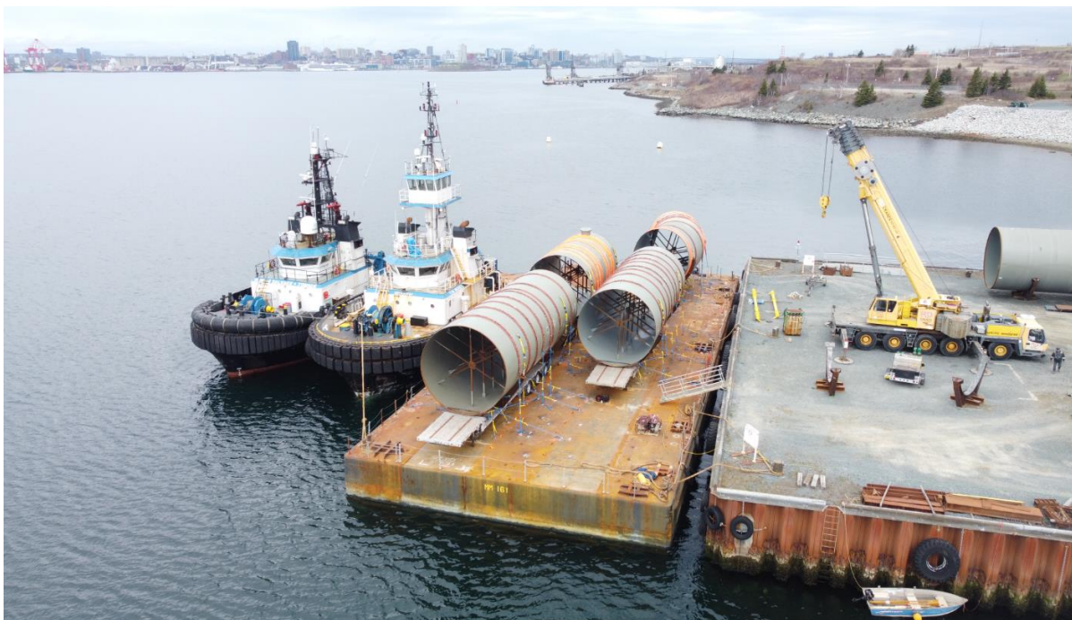
Figure 3: Barge Loadout – Cans 2,3,4 and 5
